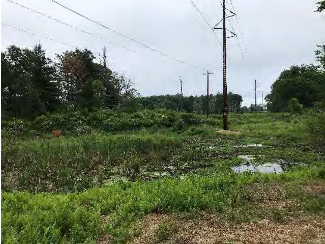
Fig 3: Str. 114 and wetland NW17. Viewing southeast. (06-22-20).
