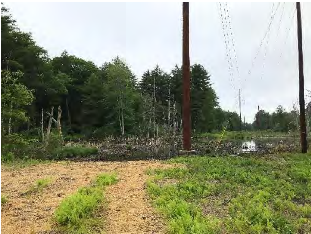
Fig 2: Str. 116 and wetland NW11. Viewing northwest. (06-22-20).
