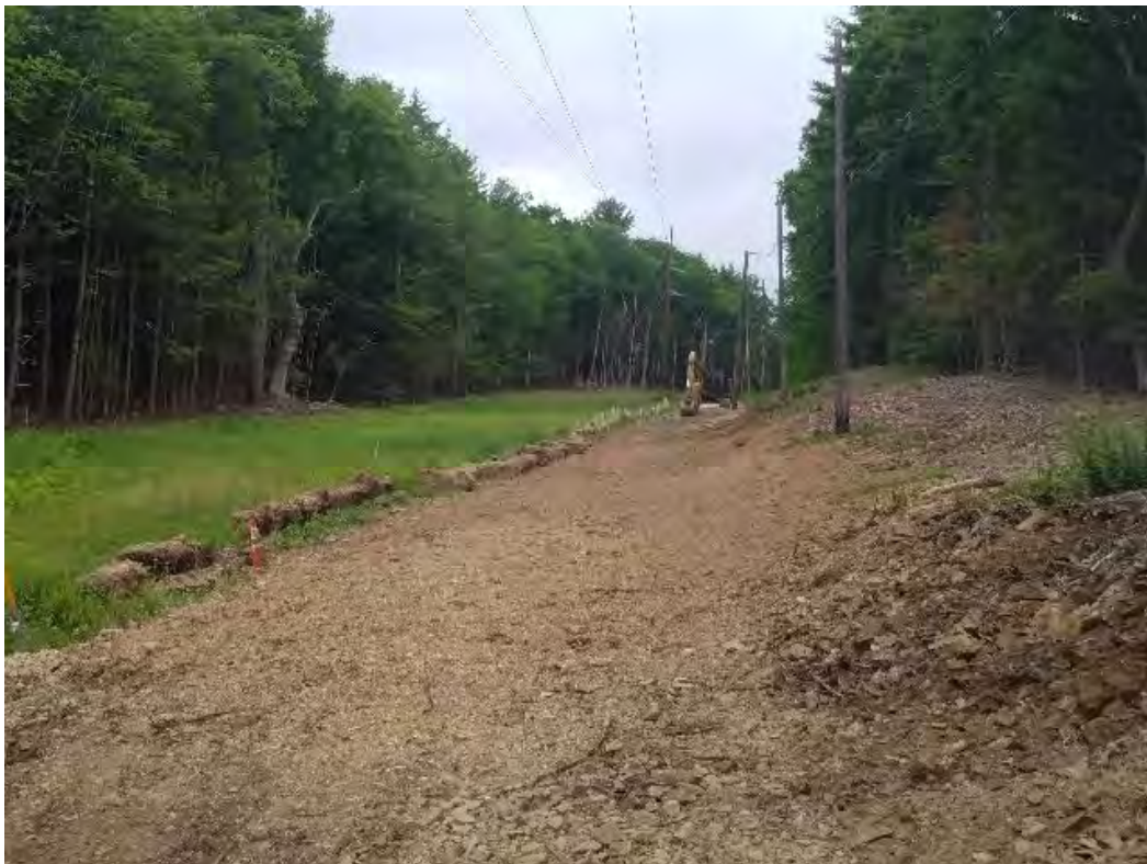
Fig 14: Crew continues to remove access road between Strs. 97-99. Viewing northwest. (06-23-20).
