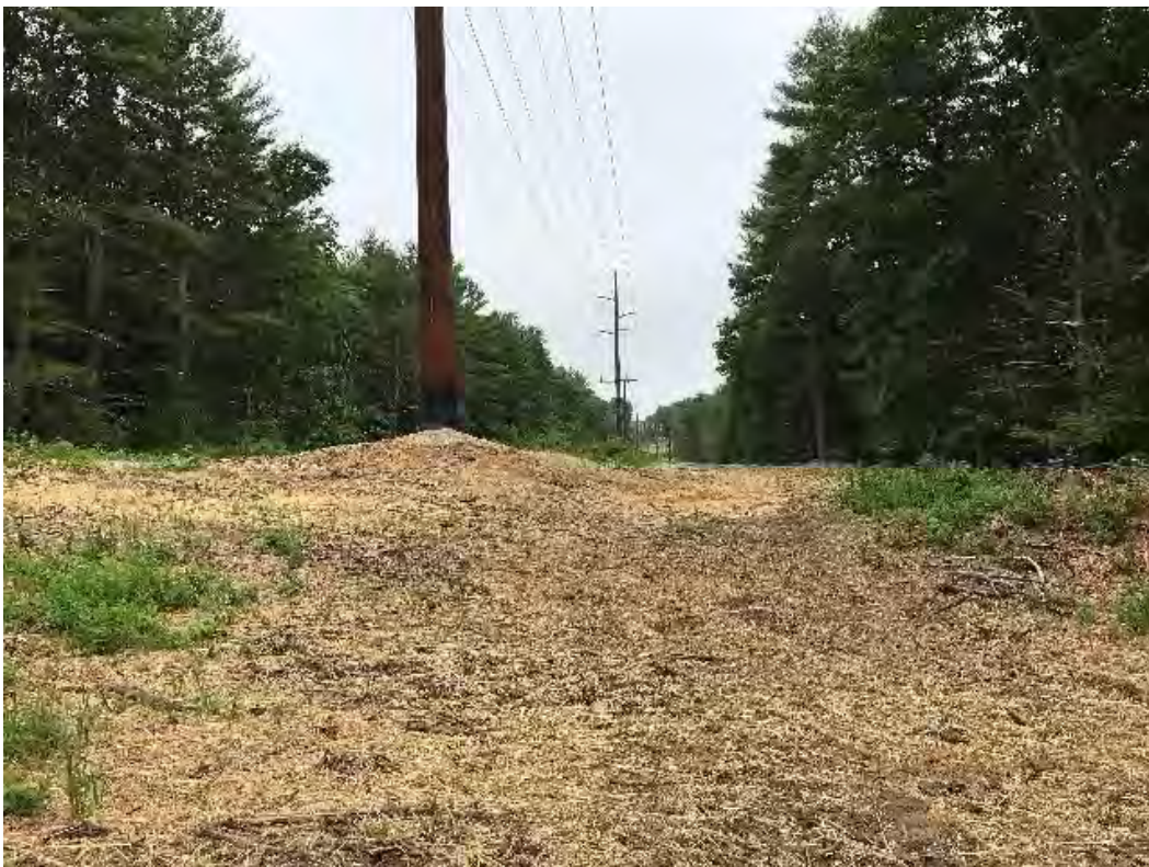
Fig 8: Str. 64 restored with some visible vegetation re-growth. Viewing west. (06-23-20).
