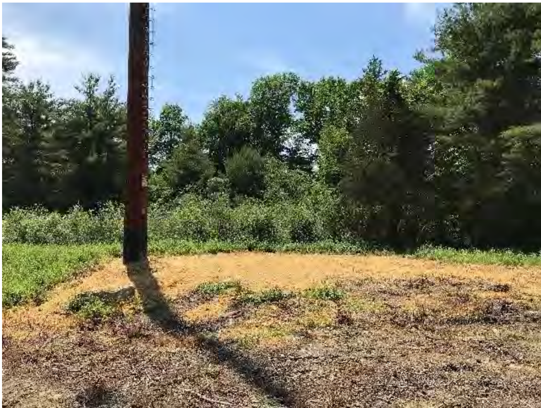
Fig 12: Str. 44 work area restored. Viewing northeast. (06-23-20).
