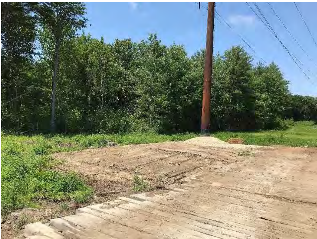
Fig 6: Crew removing timber mats used for Str. 40 work pad. Viewing northwest. (06-22-20).
