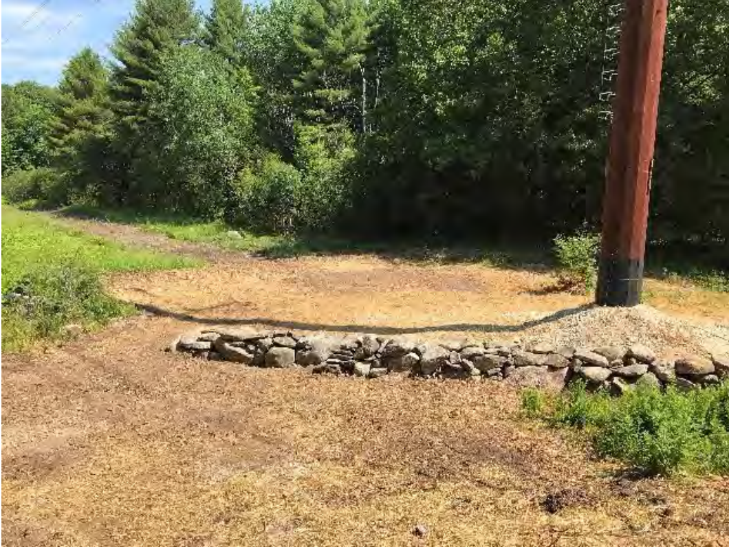
Fig 11: Stonewall WP-35 rebuilt, next to Str. 86. Viewing north. (06-23-20).
