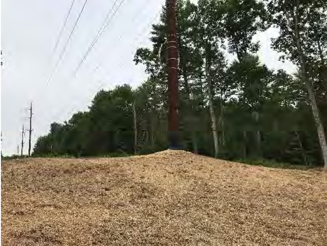
Fig 9: Str. 66 work area restored. Viewing west. (06-23-20).
