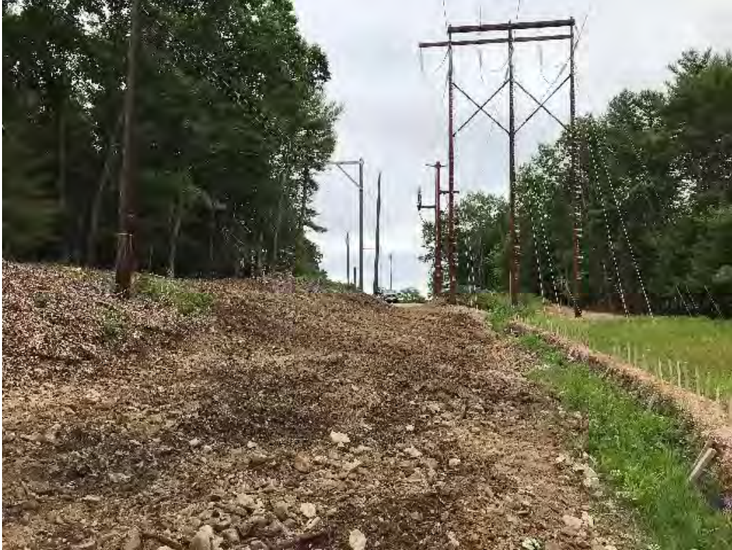
Fig 5: Crew removing access road between Strs. 97-99. Viewing east. (06-22-20).
